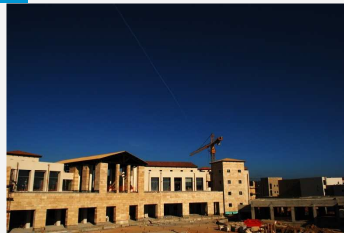
Hotel (under construction)
