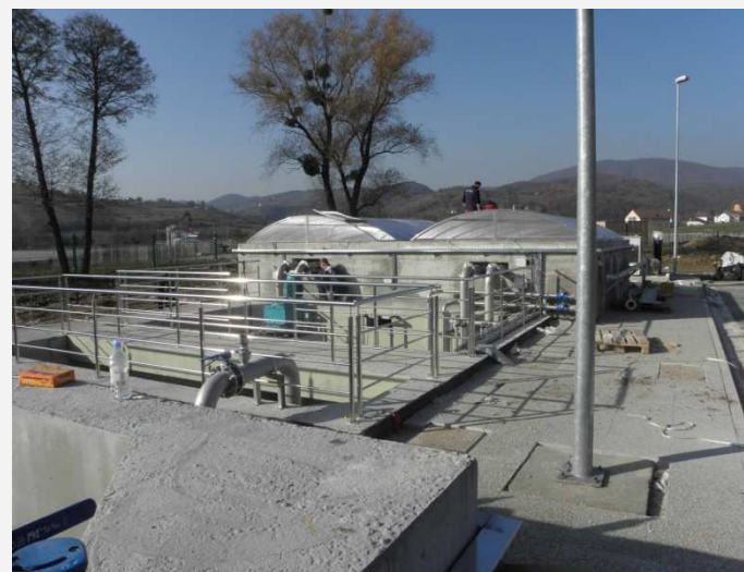
Filtration chambers (covered)
