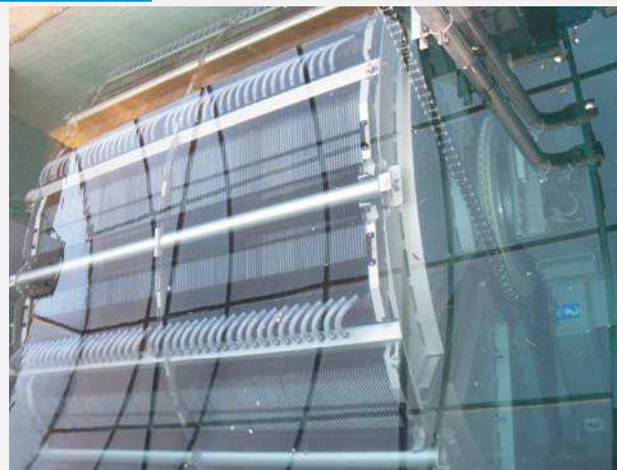
Filtration Tank before start-up
