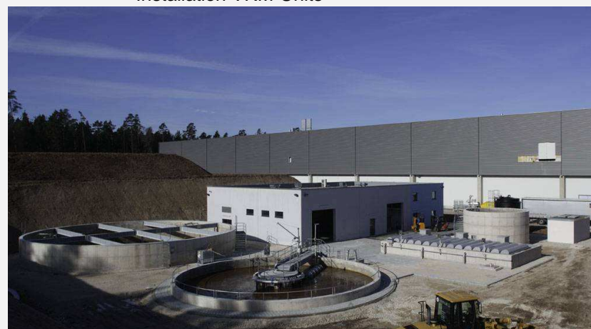
Plant overview wwtp, production plant background
