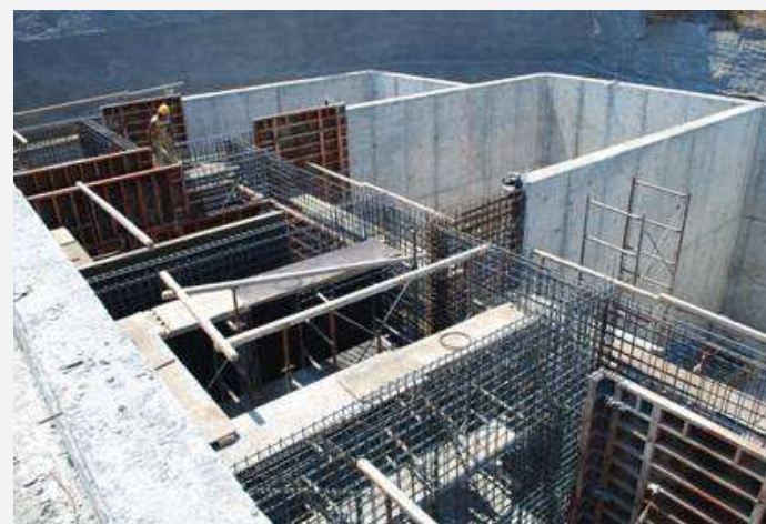
Site pictures Filtration Tanks (under construction)
