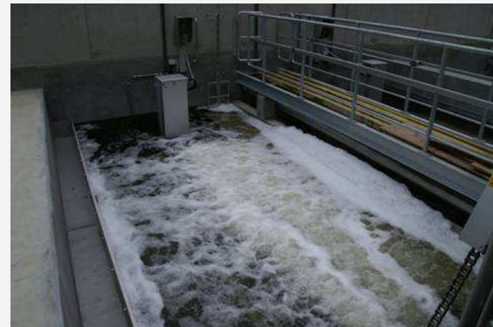
Filtration chamber, clear water test
