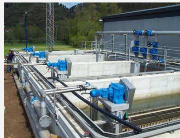
4 VRM 30/448-Units in filtration chambers
